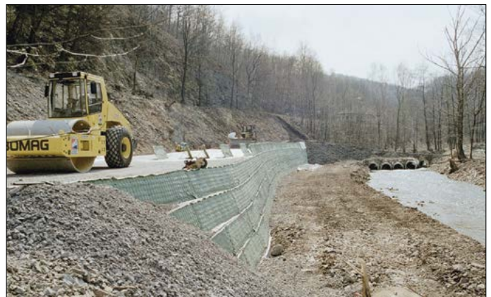
Railroad slope stabilisation
