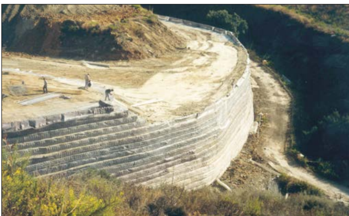
Mechanically stabilised earth (MSE) wall construction
