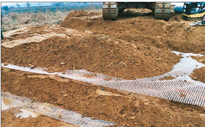
Two layers of Secugrid® as road embankment reinforcement
