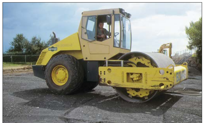
Compaction of aggregate on top of Secugrid®
