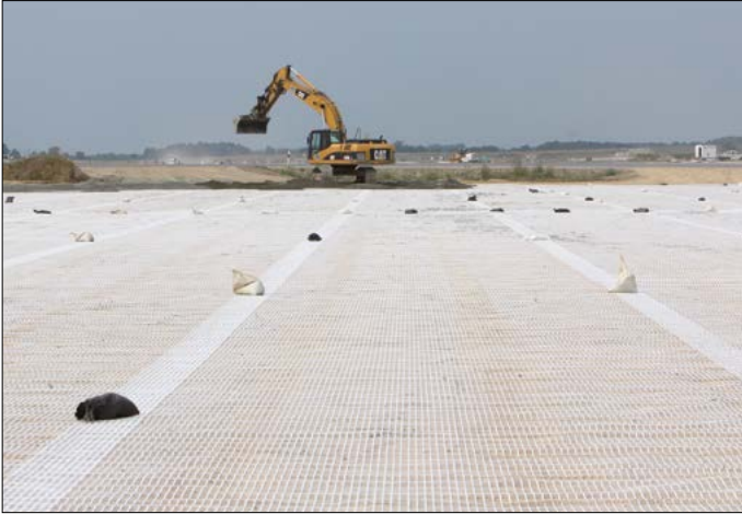
Fig. 7 Installed Secugrid® as a base course reinforcement
