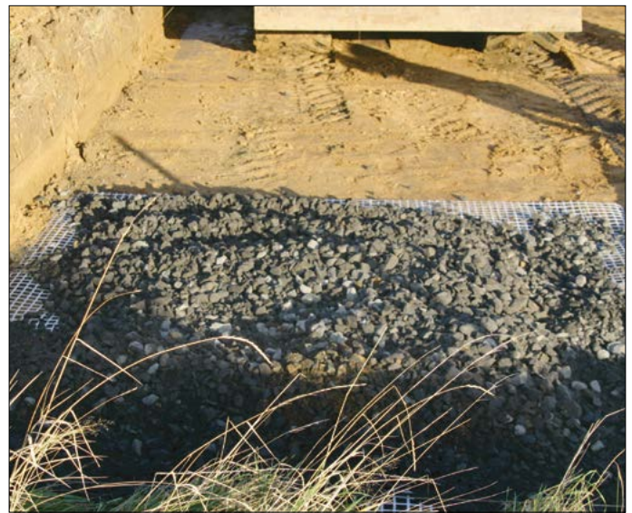
Fig. 17 Placement of base course gravel over the Secugrid® section
