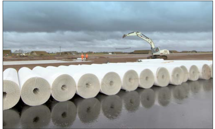
Naue Secugrid® storage on site
